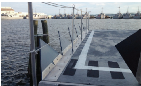
FIGURE 23. Flow control fences added starboard side of YP676 flight deck.
